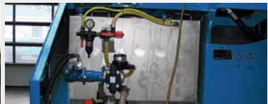
Concentrate injection tank – enzymes for fast composting
