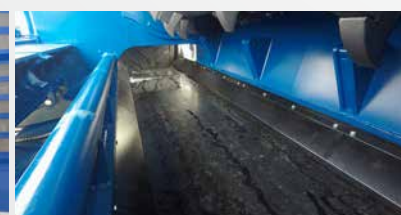
Large openings for material transport
